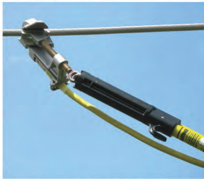
INSTALLING CLAMP
